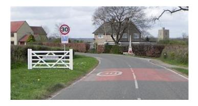
May be at one or both sides of road, various patterns and widths of gates available. May incorporate 30mph speed limit sign or parish boundary sign.
